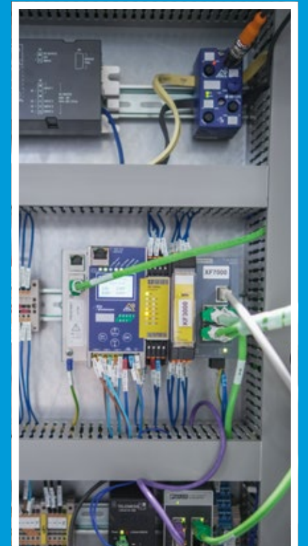
To use process data, IO-Link sensors can be easily integrated into existing ASi networks via ASi-5 Modules with integrated IO-Link Masters (above) and ASi-5/ASi-3 Safety Gateways (below) from Bihl+Wiedemann.
